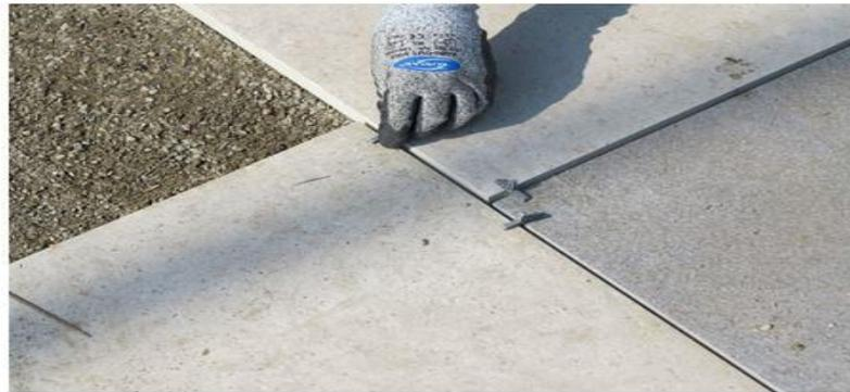
Select size and color of the pavers and install them on the prepared surface. Complete the laying scheme according to the project specifications or to your preferences.
